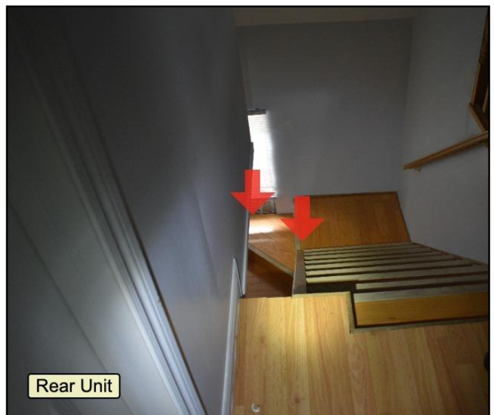
30. Missing guardrail
