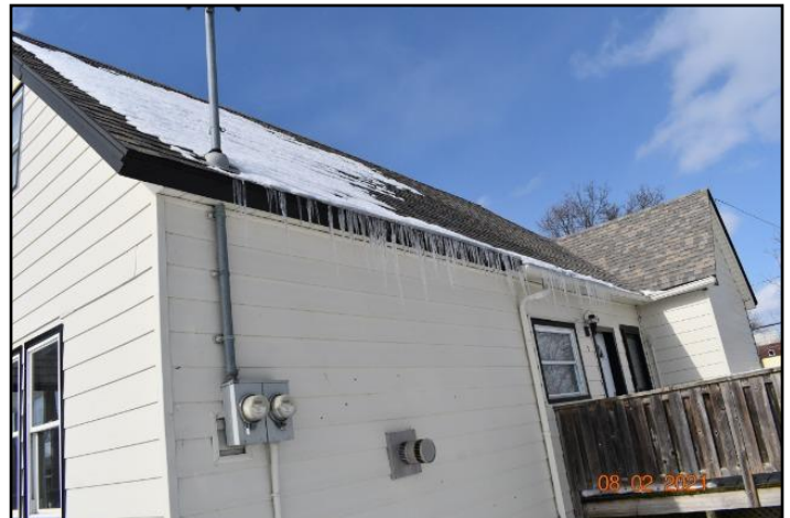
4. Missing gutters/downspouts
