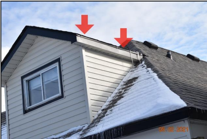
7. Missing gutter/downspouts
