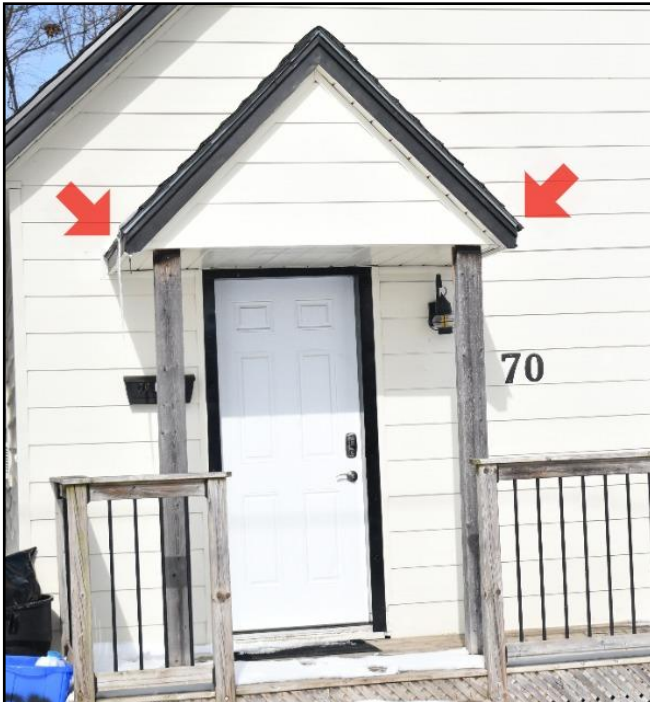
5. Missing gutters/downspouts
