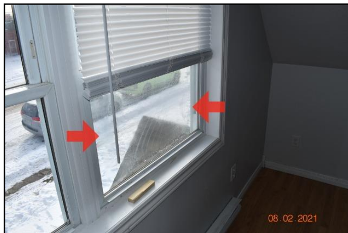
25. Lost seal on double or triple glazing
