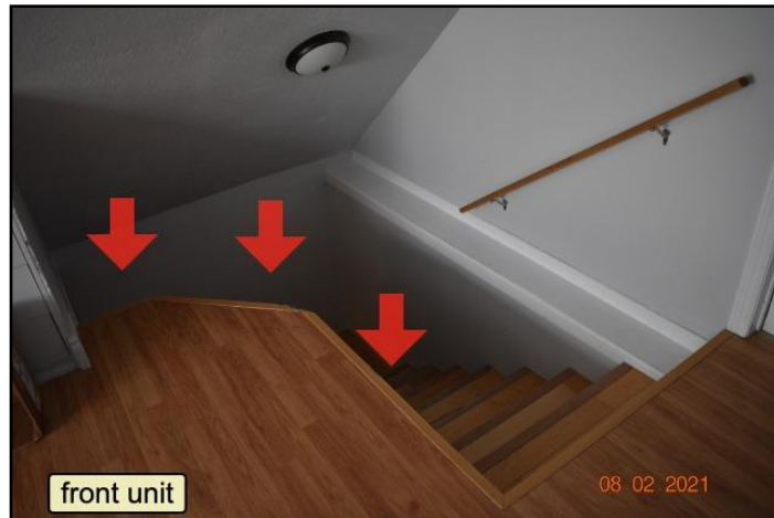
31. Missing guardrail
