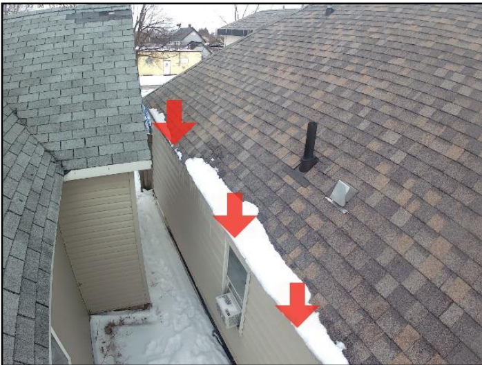
3. Missing gutters/downspouts
